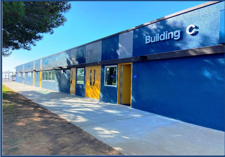
Oak Crest M.S. / Buildings. C & I Modernization
