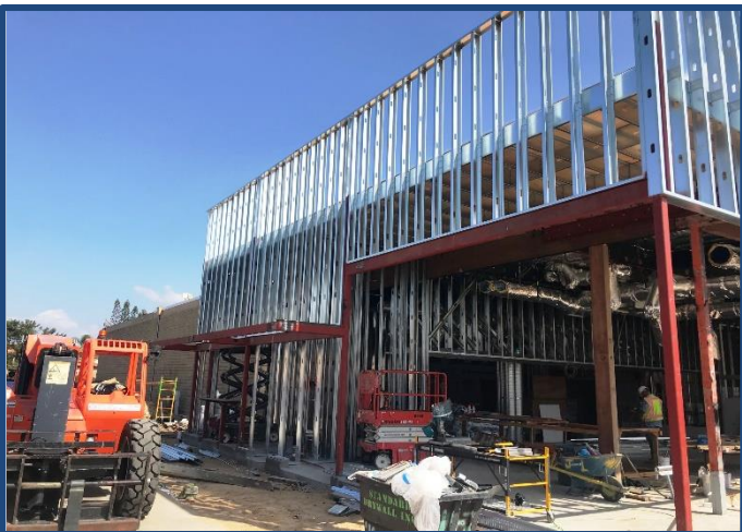
Torrey Pines H.S. / Building I
